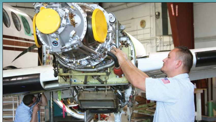
Maintenance Team Leader Shane Tuttle installs a Blackhawk Super XP 52 engine on a King Air B200
